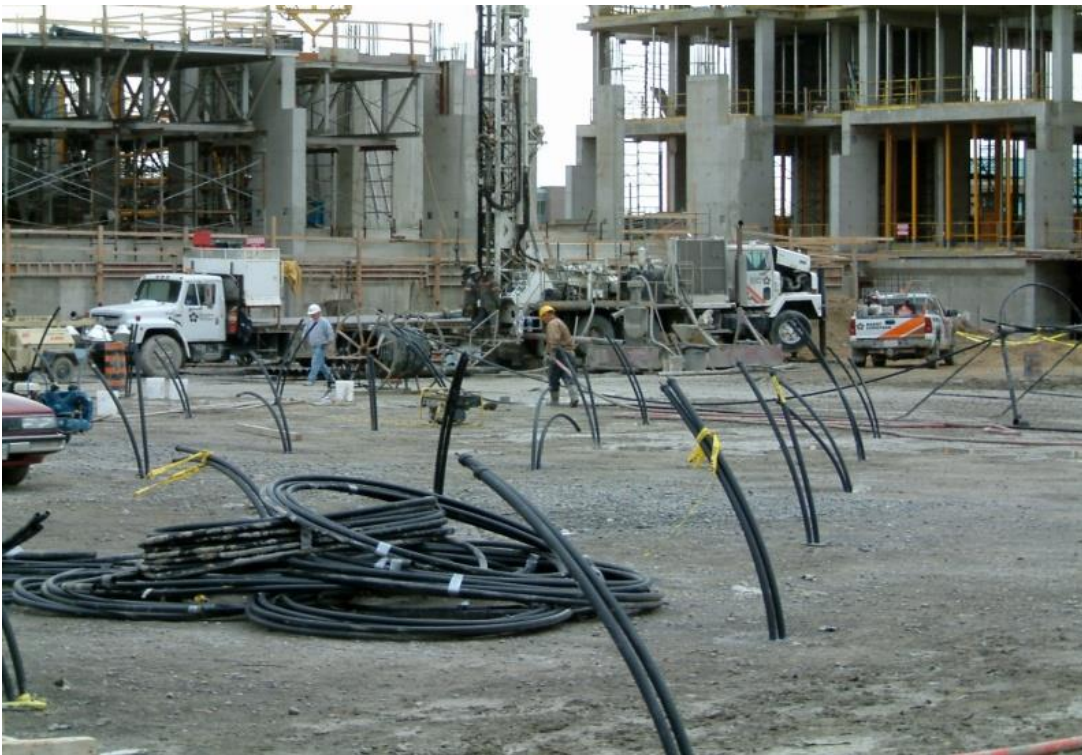
Installation of a Geothermal System (Integral Group)
