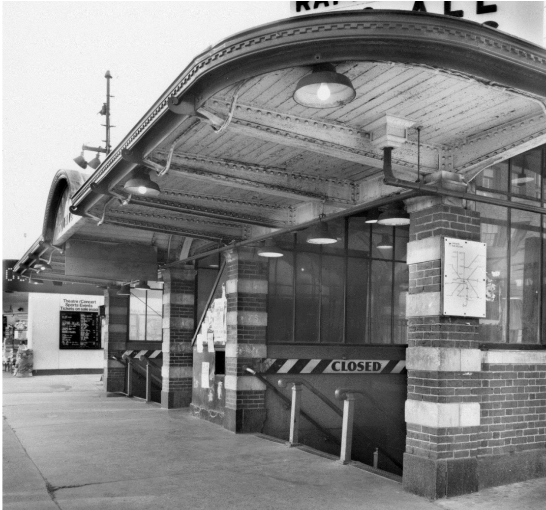
West elevation, 1977, showing roof edge dentil detail
