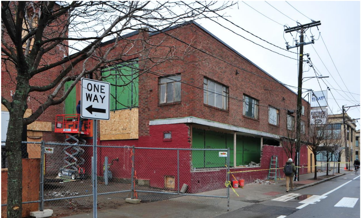
EMF Building, 116 Brookline Street, February 2019
