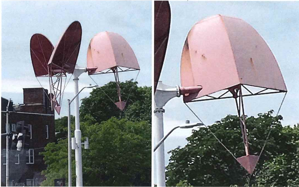
Left: sculpture showing faded paint and rust. Right: detail faded paint and rust blisters.
