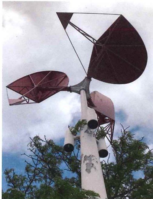
Right: flaking paint below the light fixtures.
