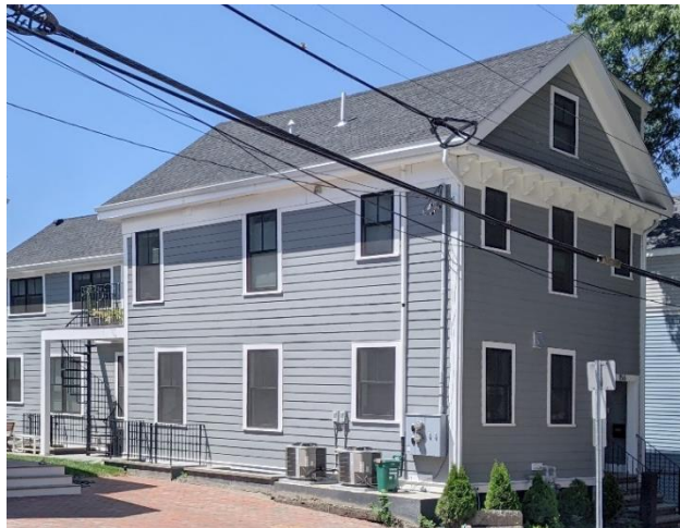
156 Thorndike Street as completed, showing removal of cornice brackets and random placement and sizes of windows. CHC staff photo, July 2022
