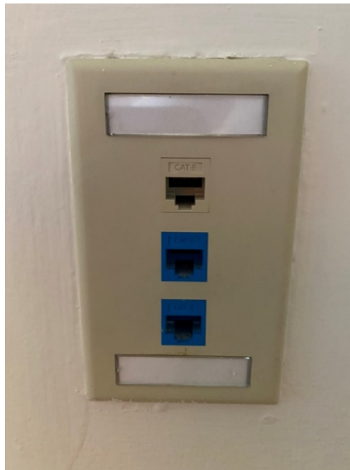
Figure 4: Ethernet Jack with Cat 6 cabling in Newtowne Court Unit
