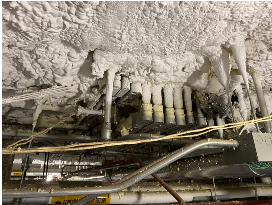
Figure 5: Spray Foam Insulation Covers Ceiling of Washington Elms Basements
