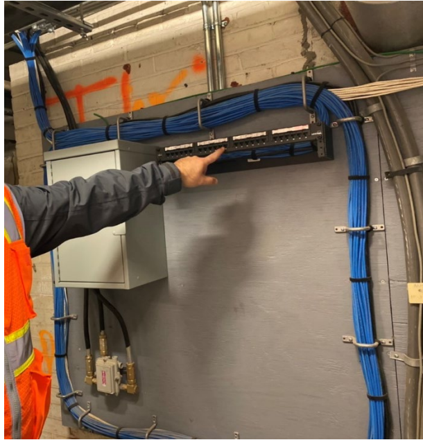
Figure 3: Cat 6 Wiring in Basement of Newtowne Court
