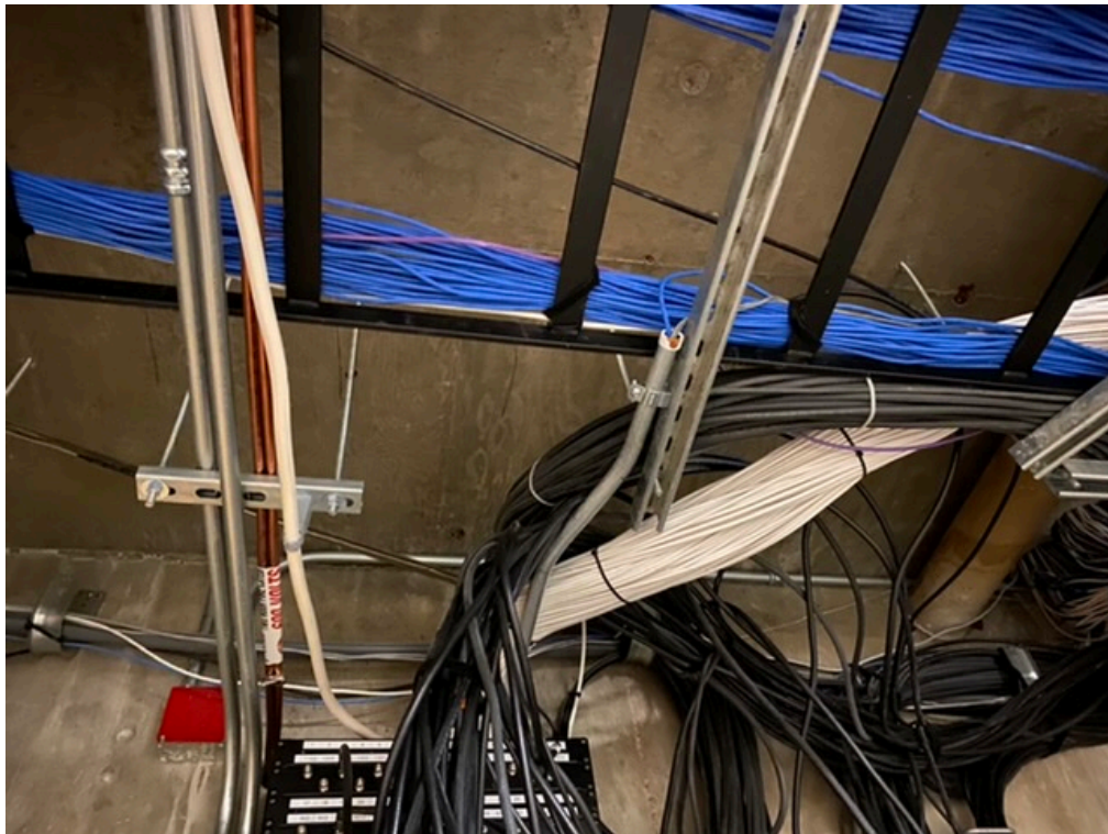
Figure 1: Cat 6 Wiring in the Basement of Manning Apartments
