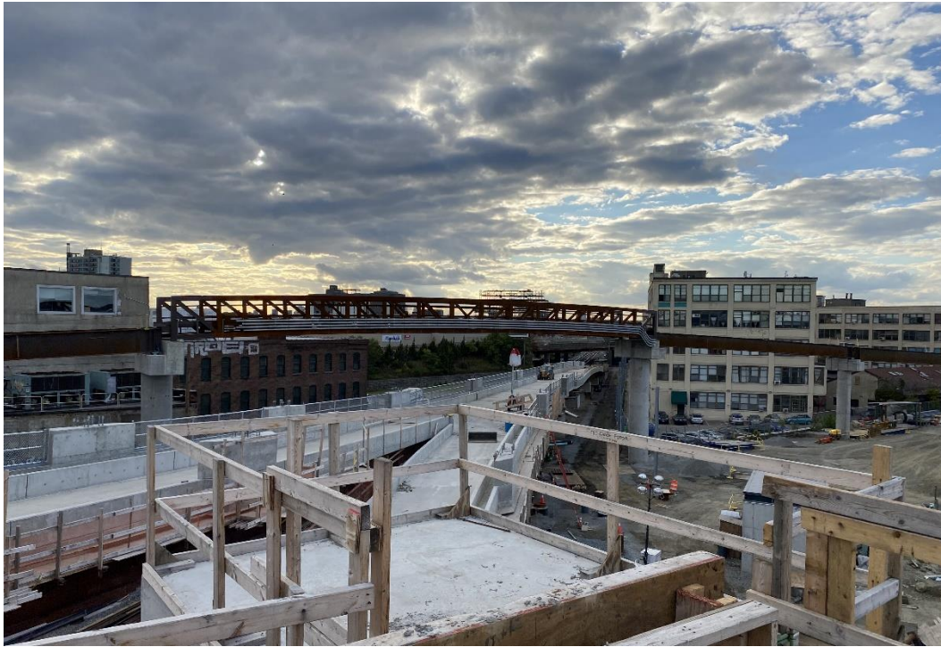
Photograph 3-View of the Community Path bridge crossing the GLX alignment heading towards Union Square (Brickbottom Artists Building on the right)
