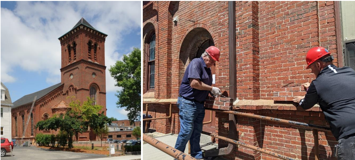
Restoration of Christ the King Methodist Church
