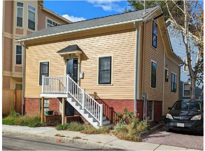
71 Bolton Street, affordable housing restored with Preservation Grant assistance
