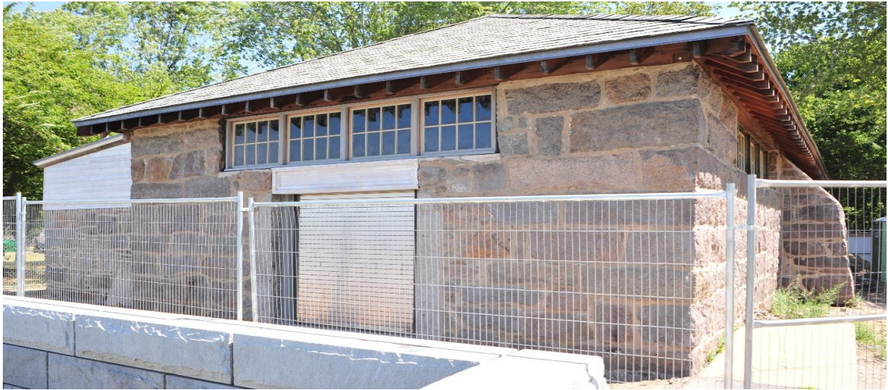
Restored masonry, with new roof, windows and security door.
