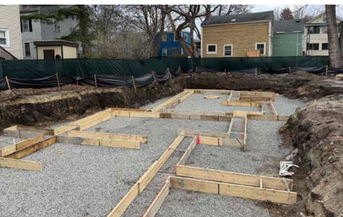
35 Cherry Street, The Port, 10 units — Status: under construction.
