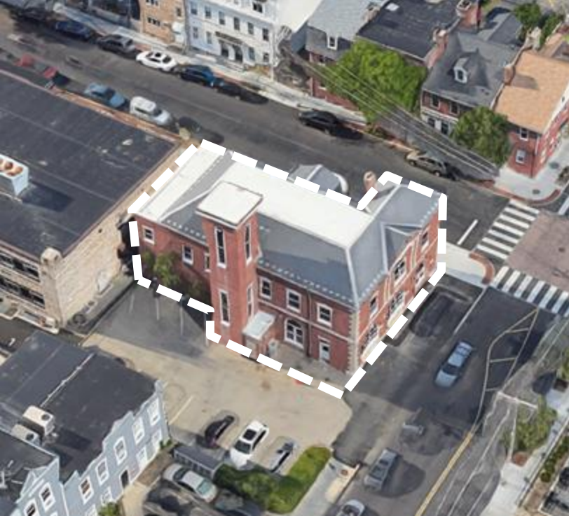
DPW ELECTRICAL (3 rd St)
