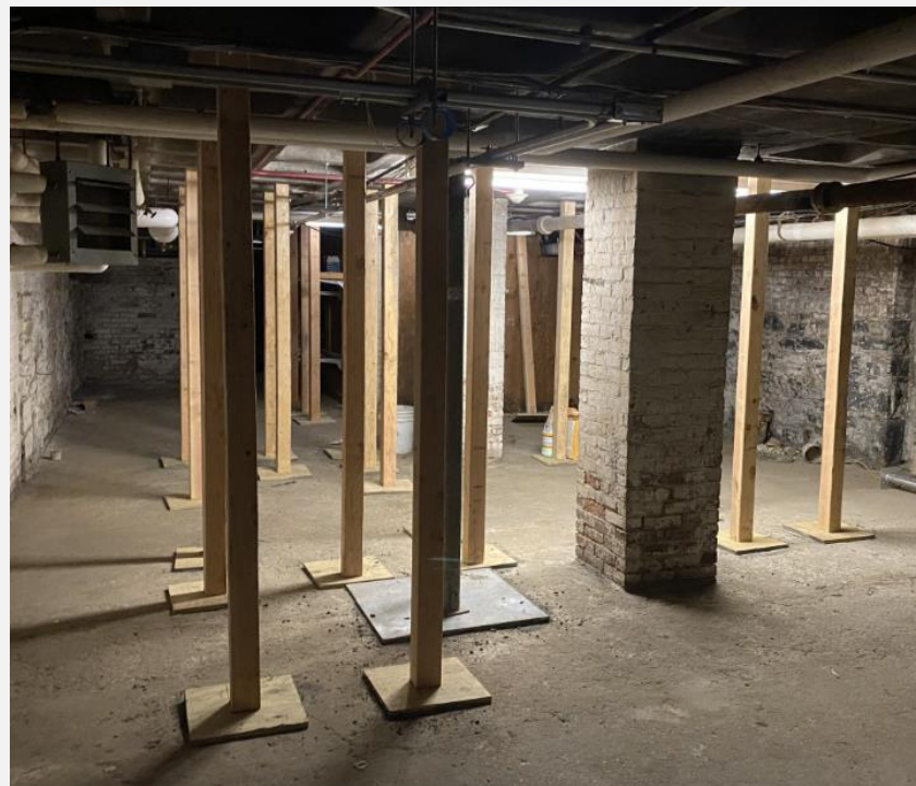
Lafayette Sq. Firehouse, critical improvements to address failing apparatus bay floor slab
