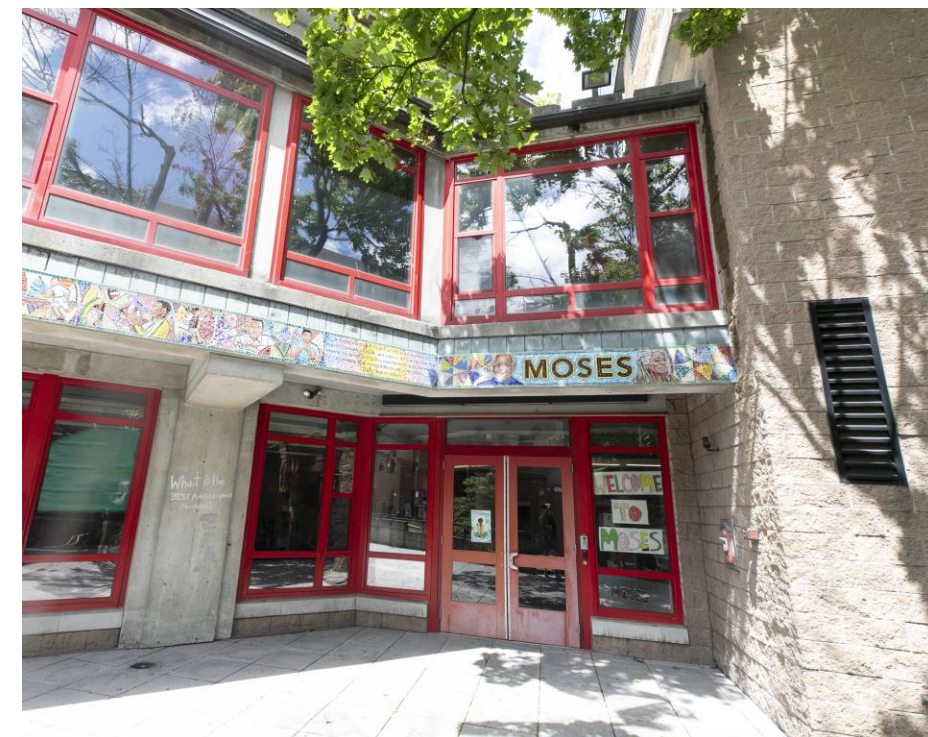
Moses Youth Center, HVAC upgrade and accessibility and plumbing improvements
