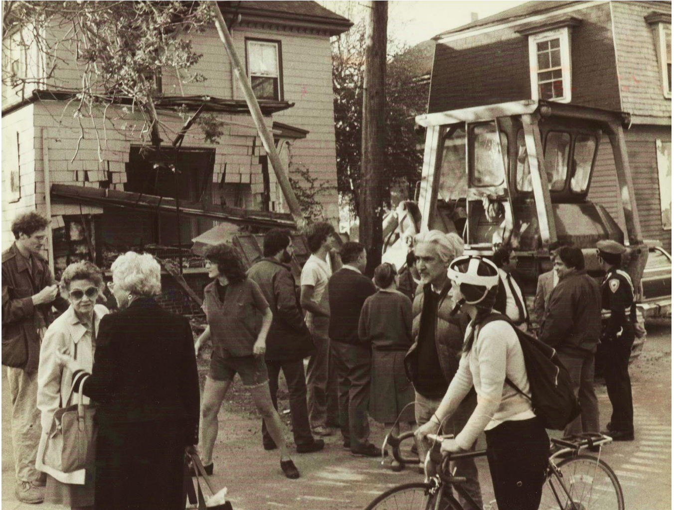
"Cambridge Residents Block Demolition of House" Boston Globe photo, May 17, 1982.
