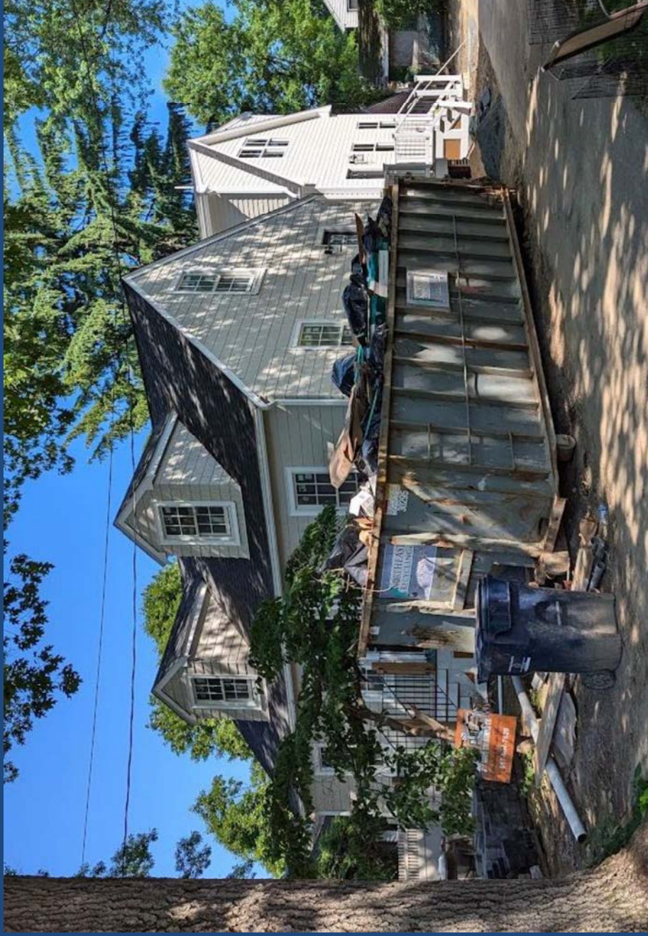
21 Loomis Street (house restored and two new units in new construction, 2023)
