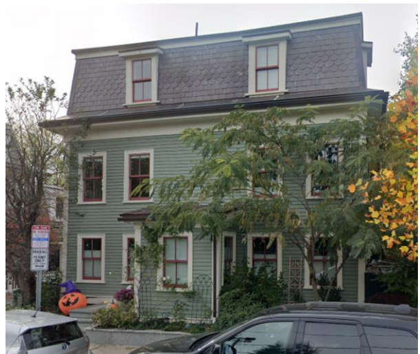
31-33 Willard Street, After (2020)
