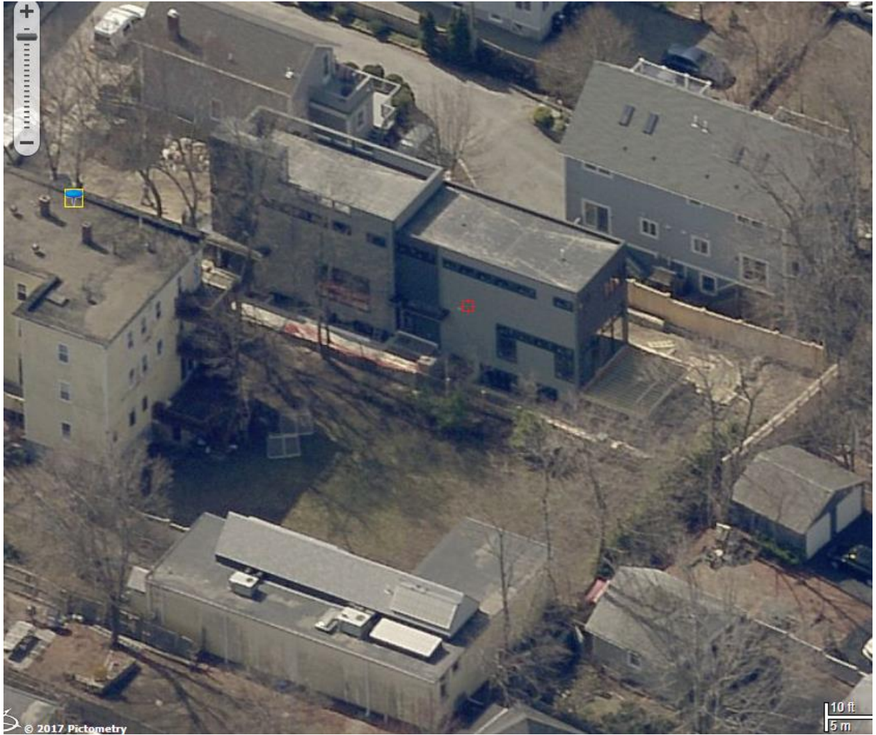
9 Donnell Street Post-Infill Project 2017
