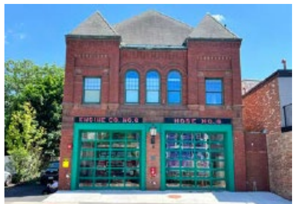
River Street Firehouse
